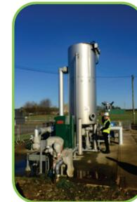
Fig. 2 Demonstration IABR located at Packington STW, UK 5m<sup>3</sup>, HRT 12 – 24h
