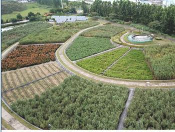
Figure 3: Tertiary treatment for water reuse. 20.000 m<sup>2</sup> vertical flow wetland.
