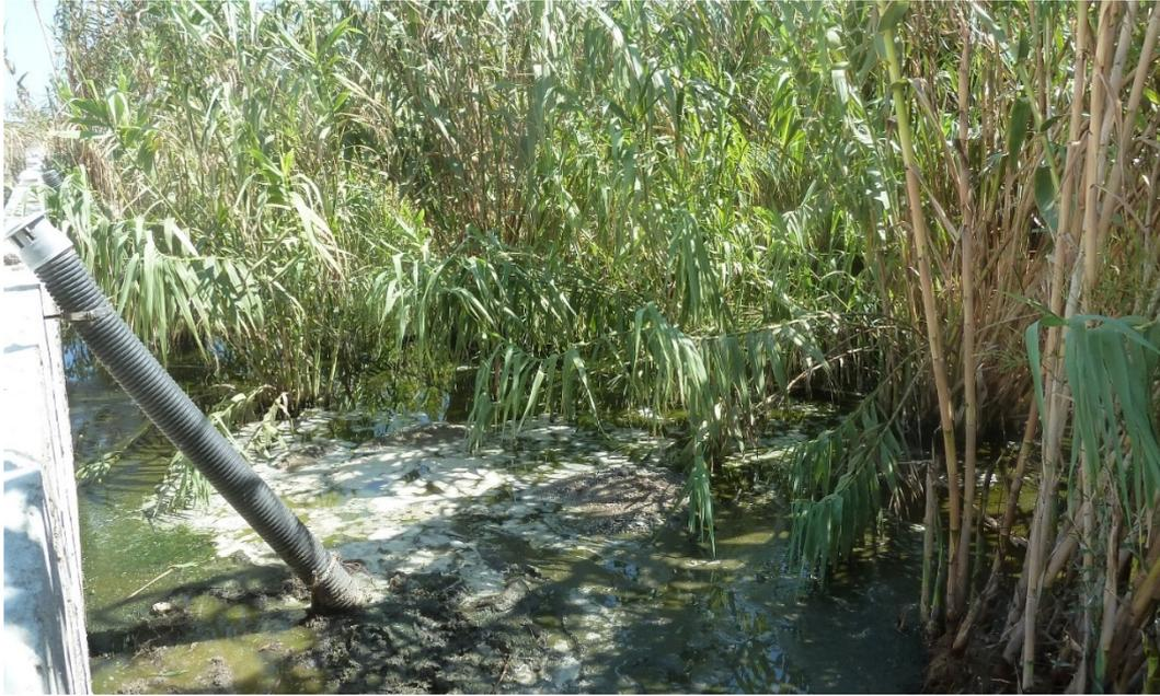
**Figure 25** Ponding in horizontal subsurface flow wetland system (16-08-2018).
