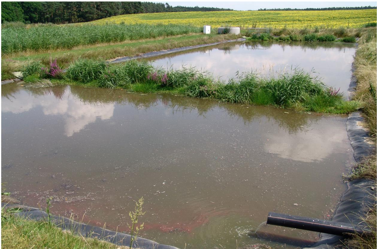
**Figure 5** Facultative pond as primary treatment with anoxic settling zone and recirculation of nitrates from VF sand filtration wetland for denitrification. Effluent from the opposite side is separated by two floating island baffles (Kappe, Germany).
