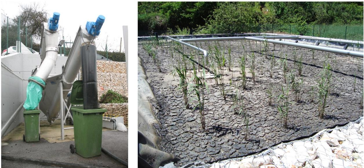
**Figure 4** Compact screen and grit trap (*KUH headworks unit KKA, Aveleira, Portugal*) (left). Raw sewage distribution and filtration at 1<sup>st</sup> stage of a “French system” (*Aveleira, Portugal*) (right).
