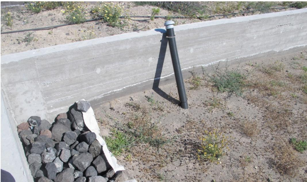
**Figure 26** High density geotextile for separating rocks/ sand and visible intrusion of salt into concrete wall from sea sand used in the filter.
