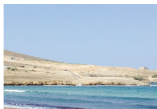
View of the WWTP
